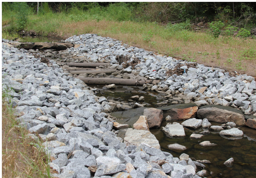
Joe's Branch Phase II Restoration
