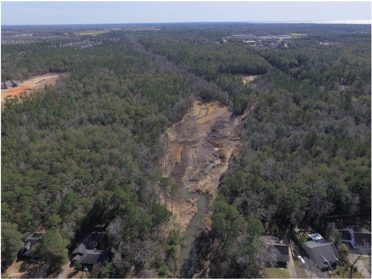
Tiawasee Creek Restoration
