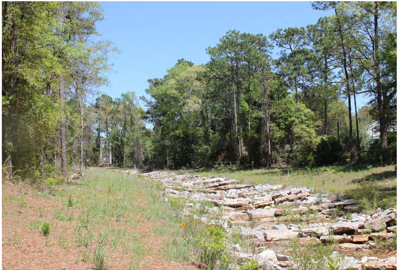
Completion of Joe's Branch Restoration.
